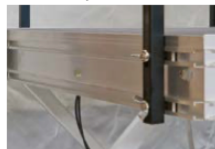
Bridage garde-corps / Handrail fixation
